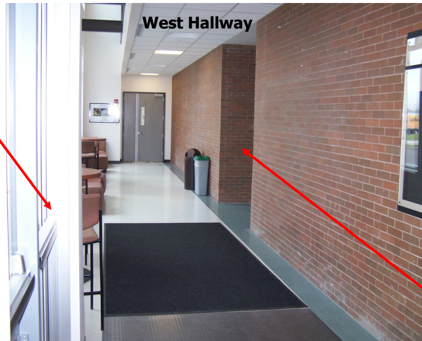
Building 17 West Exit
