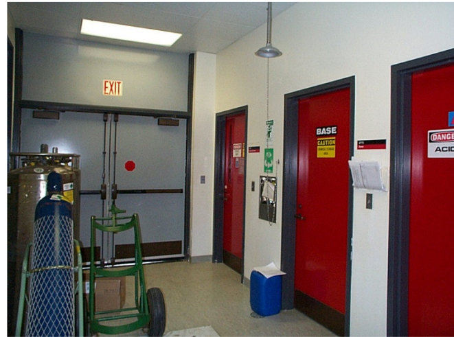
In Northeast vestibule near chemical storage
